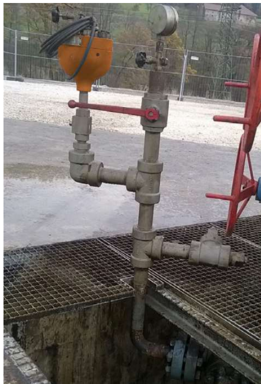
Graphic: Connection Pipework for mounting the High Pressure Sensor Unit / Transducer (Example Picture only)
